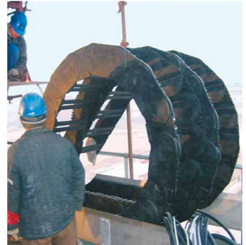
Assembly of an E4 e-chain® series 800 in a steel guide trough
