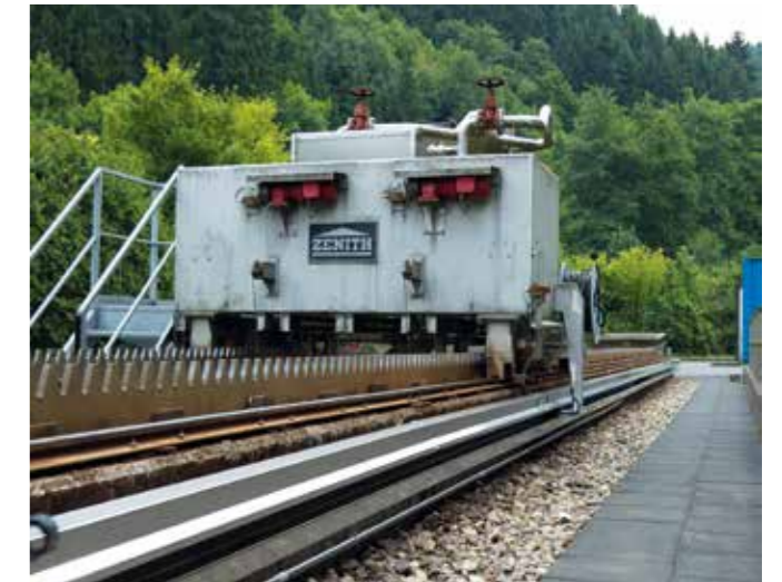
Sewage treatment plant in Volmetal, Germany - travel 26m
