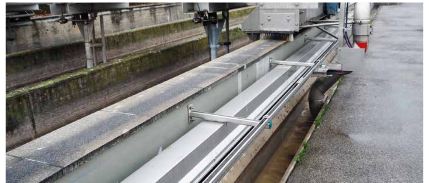
Sand traps, sewage plant in Bamberg (Germany) - travel 26m
