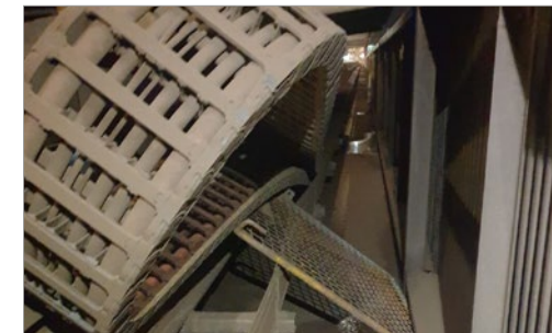
Immediate emergency shutdown by i.Sense prevents total failure
