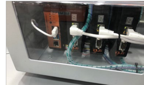
Avoid unplanned downtime through intelligent energy chain monitoring
